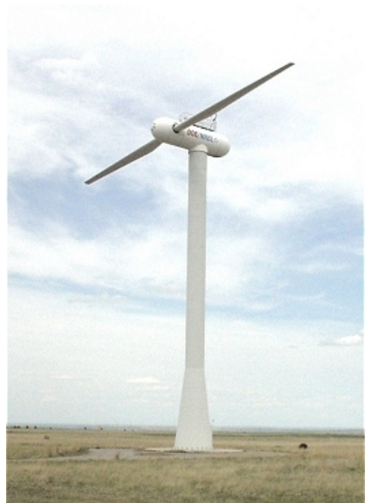
600 kW utility-scale Advanced Research Turbine at NREL's National Wind Technology Center near Golden, CO, USA. Note how the variable-pitch blades are positioned so they can't make power—the turbine is shut down and can't spin. Photo by the author.
