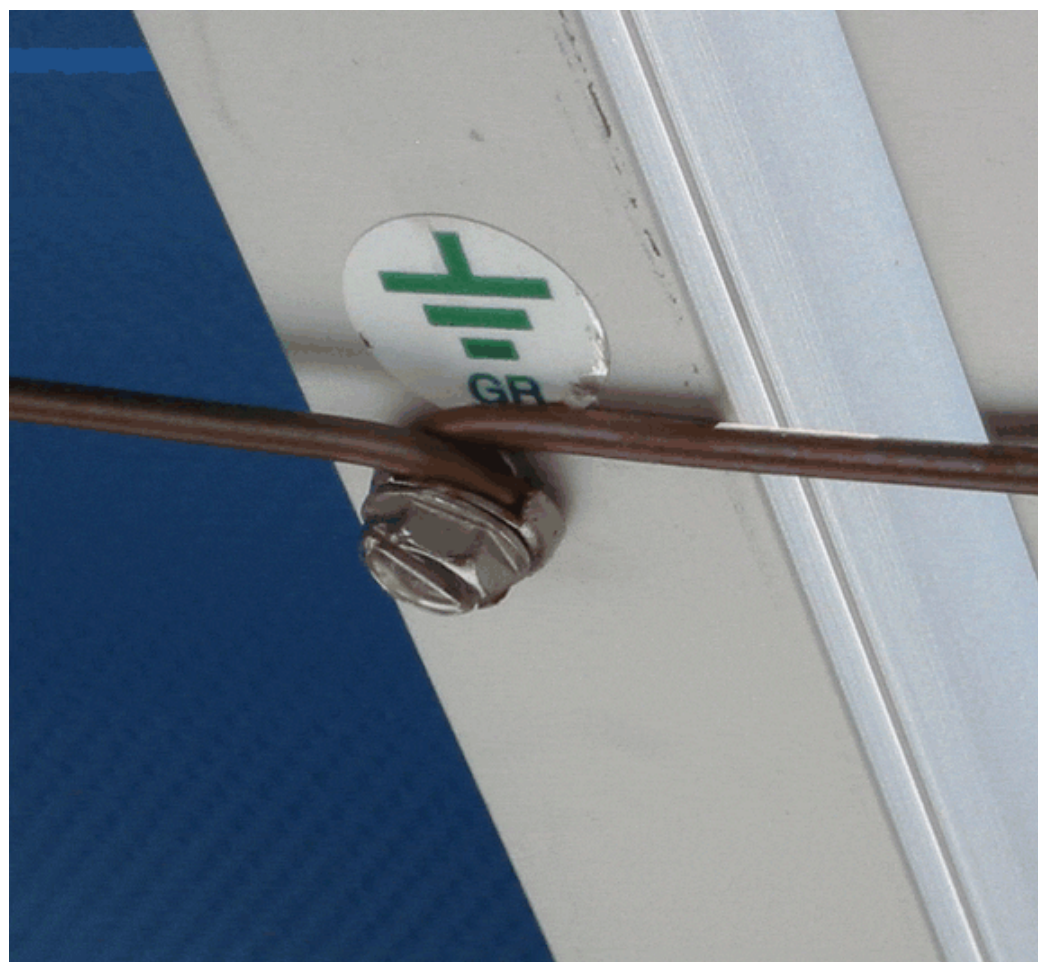
Figure G-2. Improper Module Grounding
