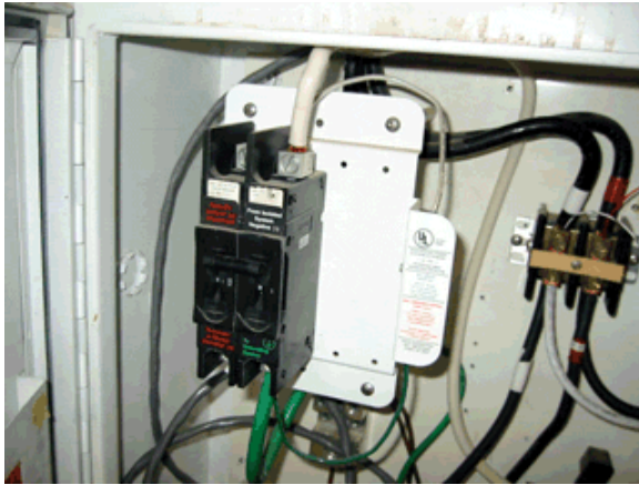
Figure 12. External Ground-Fault Protection Device
